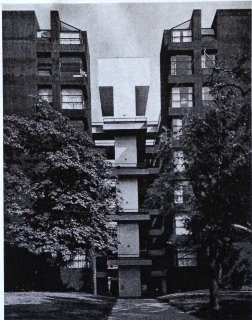
3, near view of eight-storey flats, showing two slabs linked by lift tower clad in white tiling. 4, distant view of the same, looking along the 'processional way' from the Heath to the tower.
