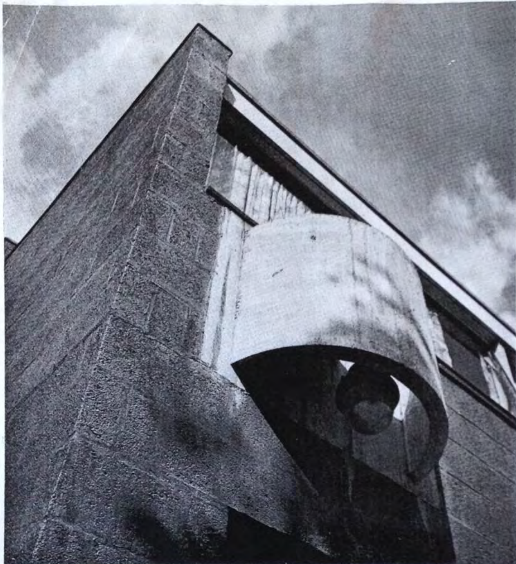
15, detail of concrete shade to light fitting. 16, interior of living room in three-bedroom house, showing central stove and chimney in staircase well. 17, same view of four-bedroom type, showing stair up from basement immediately behind stove.
